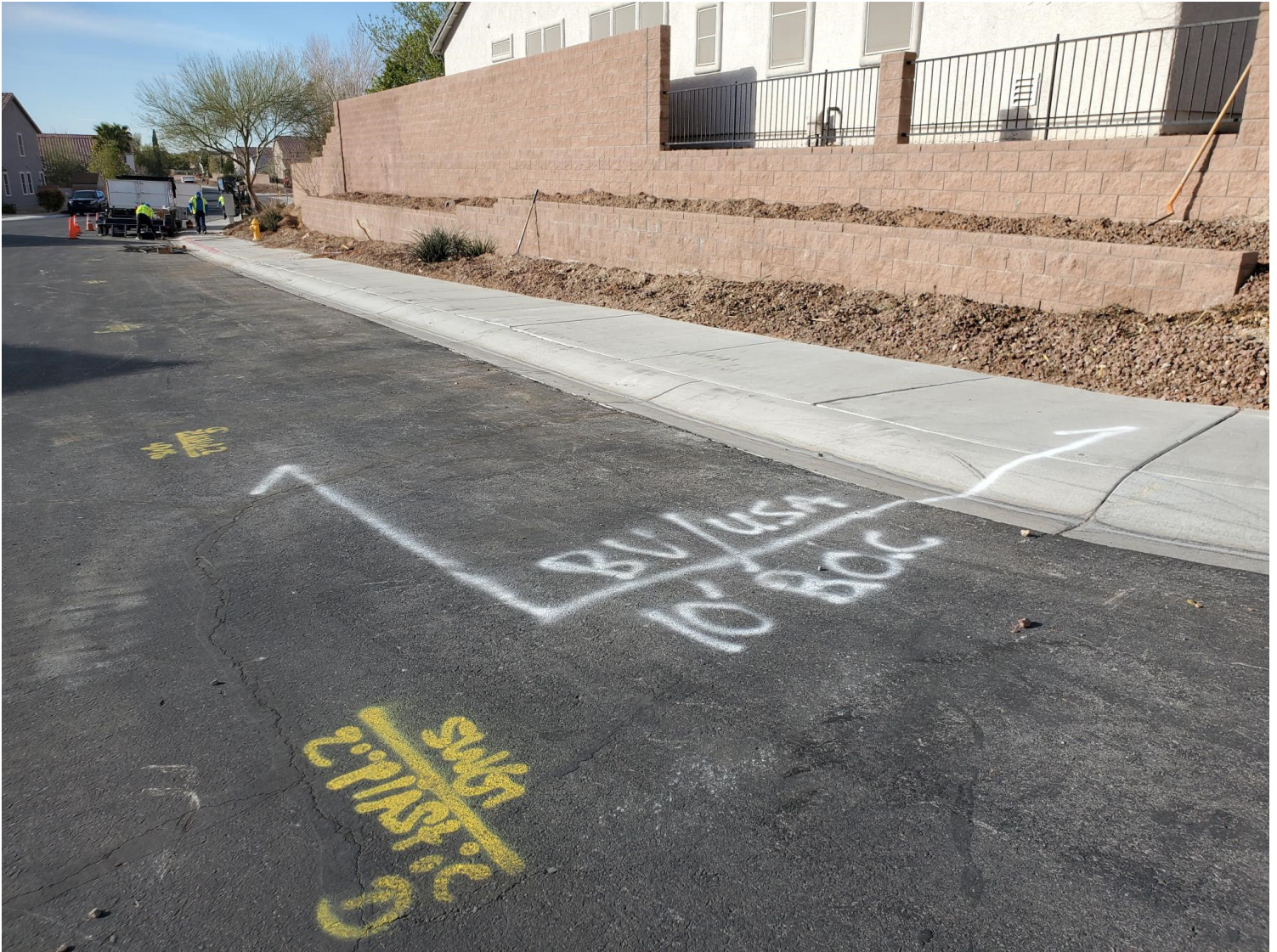
White paint marks a planned excavation in a Las Vegas neighborhood. A Southwest Gas locator marked the location of underground gas pipeline with yellow paint.
