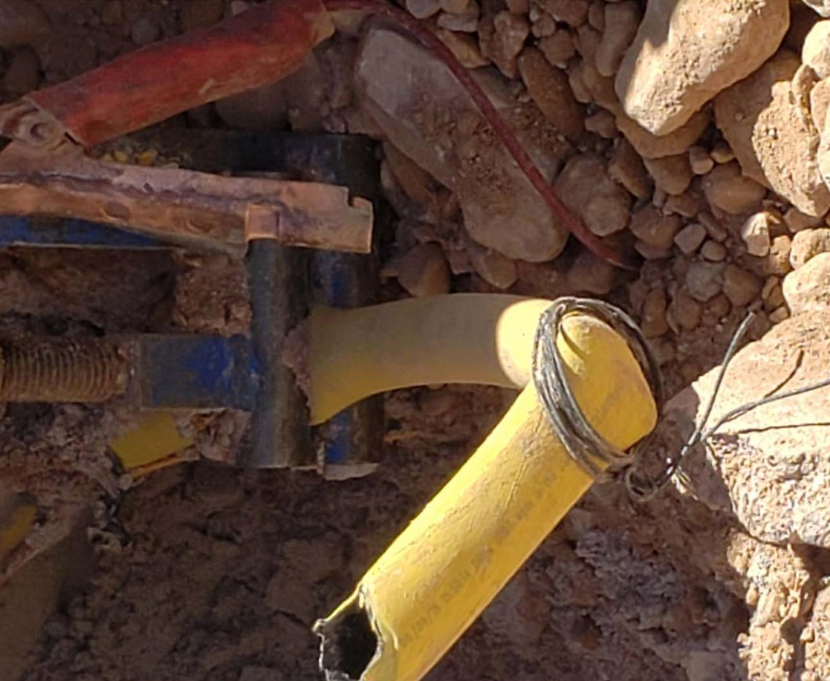
The PUCN's Pipeline Safety Program involves the inspection of jurisdictional liquid propane and natural gas piping systems statewide. In the above photo, PUCN gas pipeline engineers responded to a report of a gas pipeline damaged by an excavator. The excavator had folded over and tied the pipeline with wire in an attempt to stop the flow of gas, which is a violation of NRS Chapter 455 - Excavations and High-Voltage Lines.
